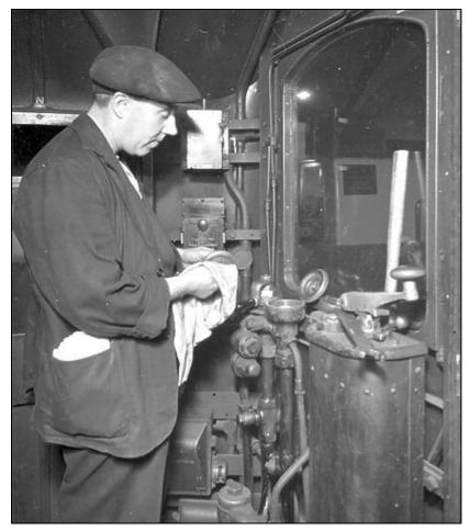
Figure 4: A fitter at Northfields Depot in September 1937 cleaning the equalising valve piston of a Westinghouse No. 4 brake valve in a control trailer cab. We can see it is a control trailer by the shape of the cab door and by the position the control switch next to the brake valve piping. The evidence of this photo suggests that not all Piccadilly line control trailers had e.p. brake controllers, even though the cars were fitted with e.p. brake operating valves. Photo: LT Museum.
